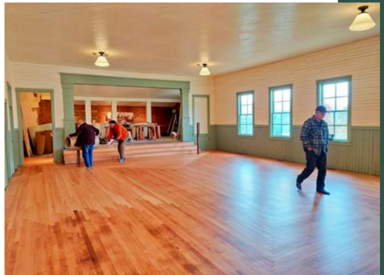
The new floor.
