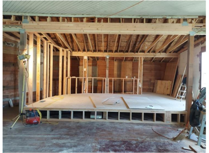
Stage is framed and ready for finishes!
