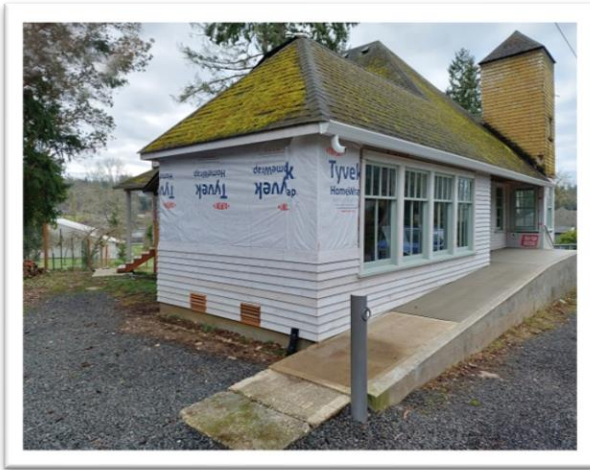
Siding progress + new historic hitching post!
