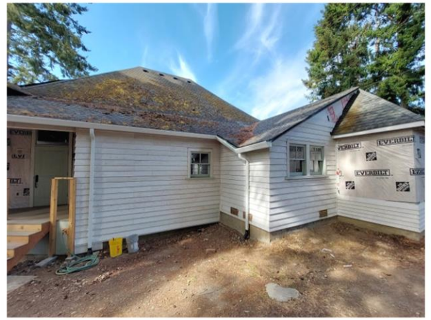
First lap siding installed, primed & ready for final paint!
